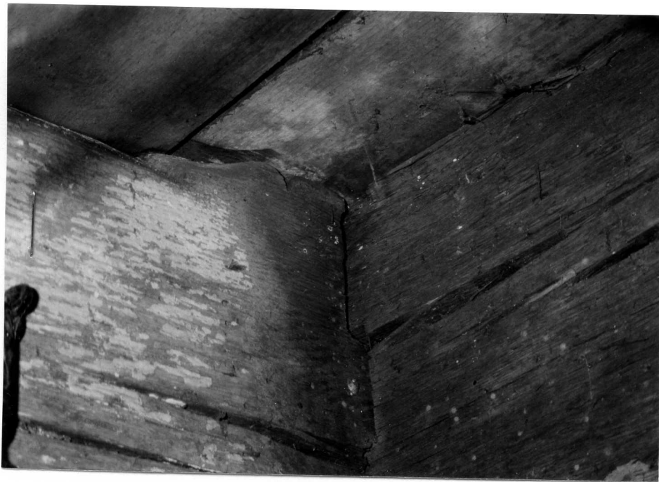
CELLAR : CHAMFERED BEAM USED AS SUPPORT TIMBER - MORTISED INTO SILL (RECYCLED)
