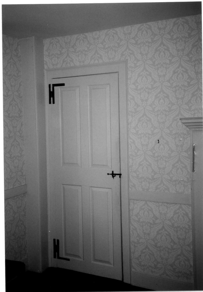
ROOM 5, FIRST FLOOR H-L HINGES AND BOXED BEADED CORNER POST
