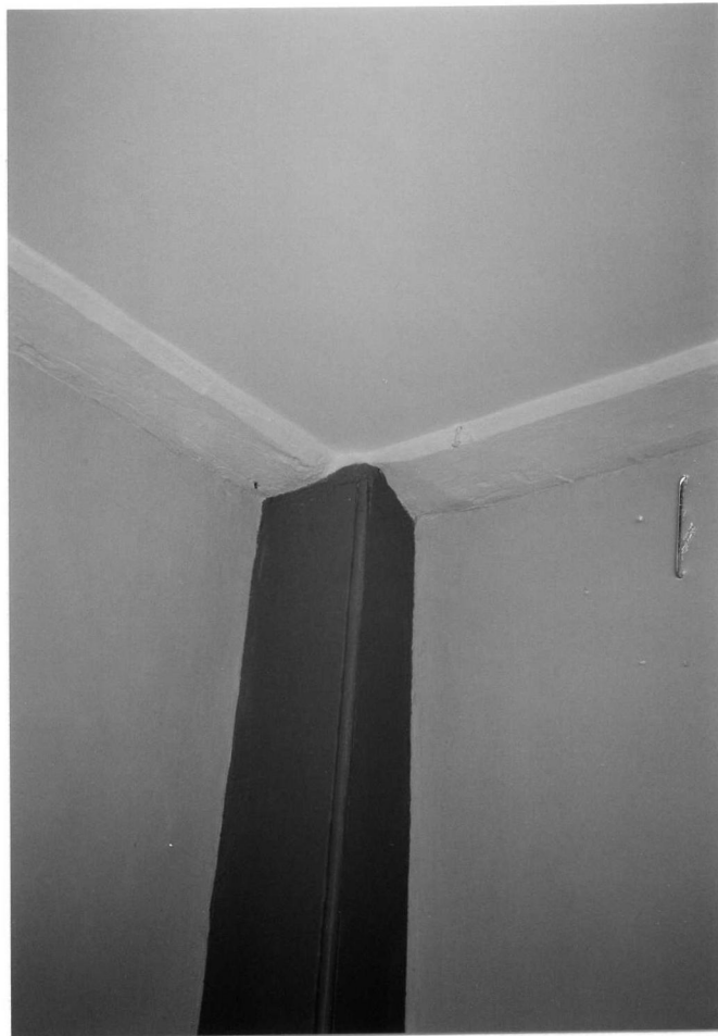
ROOM 2, FIRST FLOOR PLATE, GIRT & BOXED AND BEADED CORNER POST
