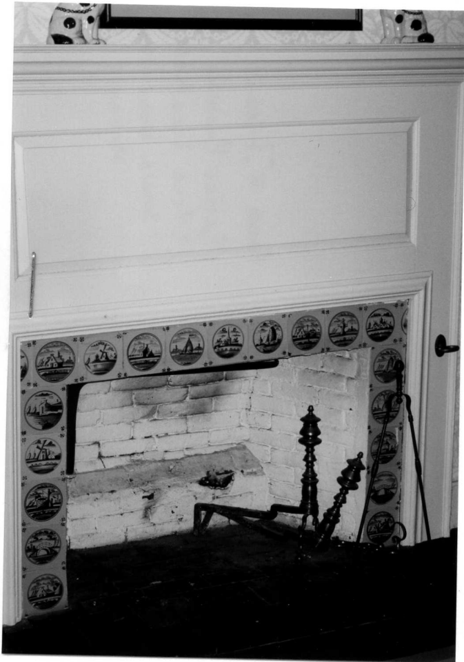
ROOM 5, FIRST FLOOR RAISED PANEL FIREPLACE SURROUND WITH TILES SMALL BOLECTION MOLDING
